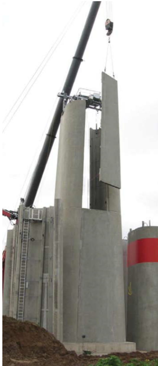
Figure 2-9: Advanced Tower Systems hybrid tower. (Vries, 2009)
