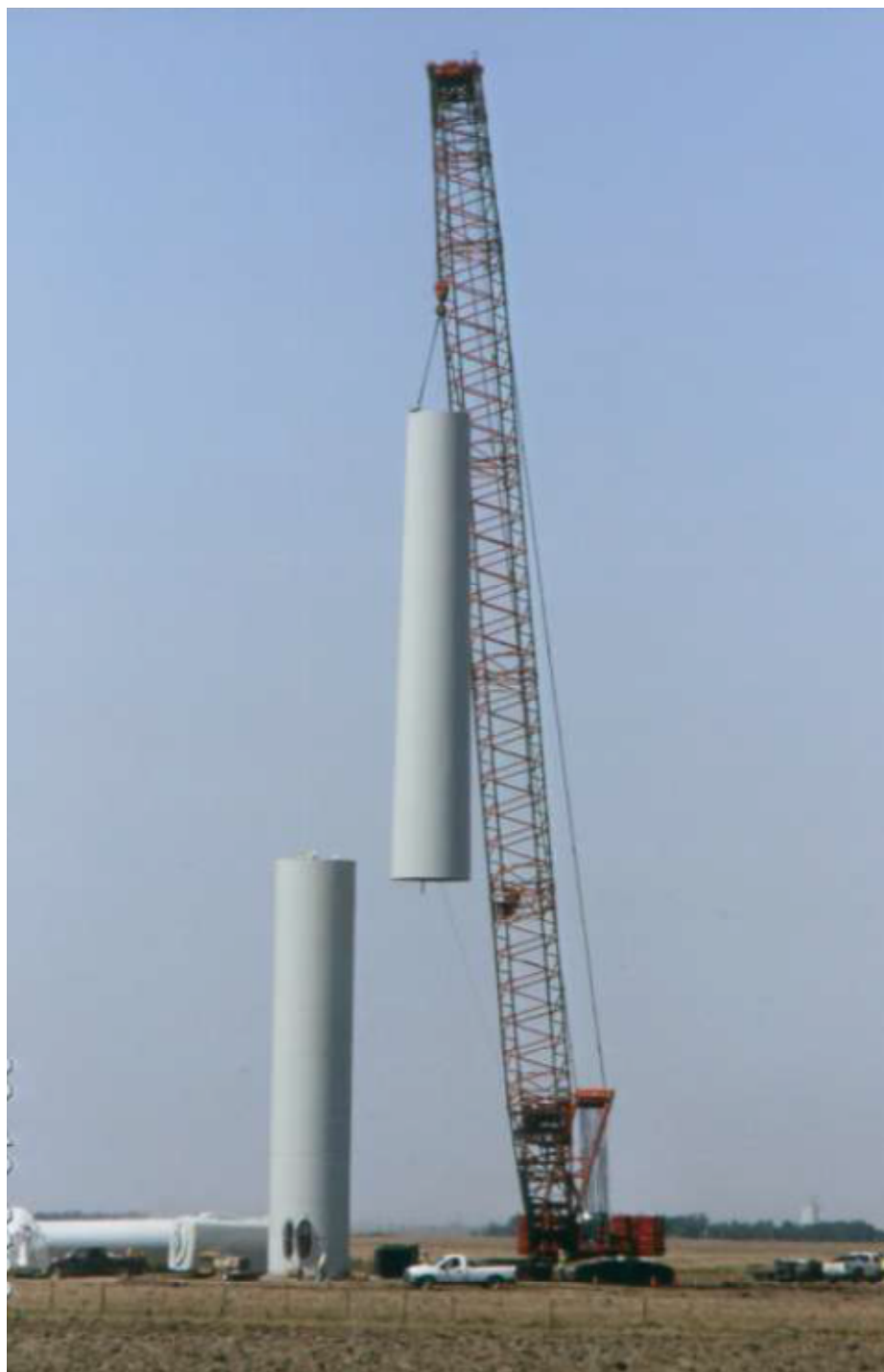
Figure 2-5: Erection of steel towers. (Sri, S., 2011)
