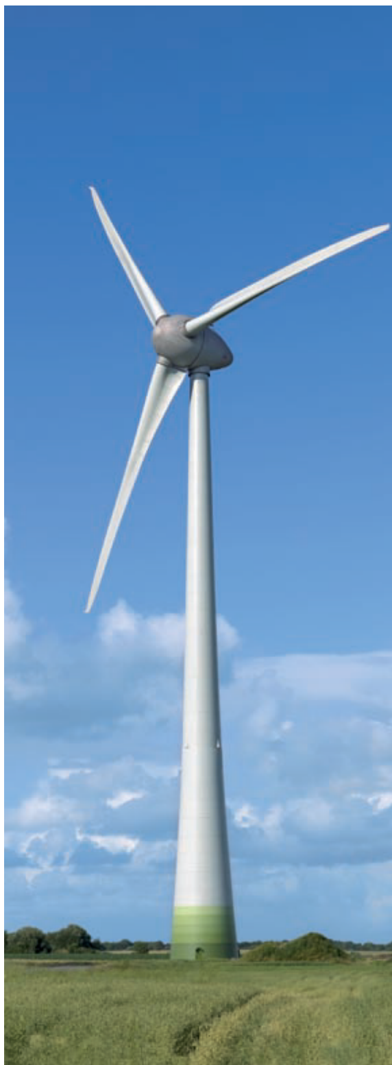
Figure 2-11: Enercon wind turbine with rated power 7.5MW. (Enercon GmbH)
