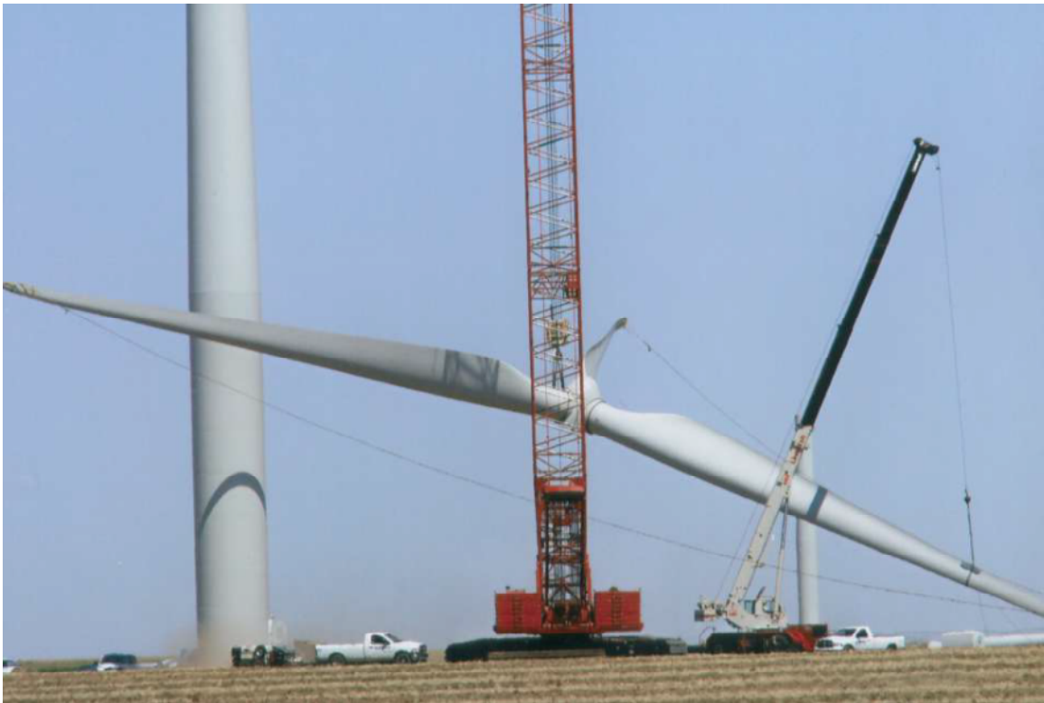
Figure 2-7: Blade tipping using two cranes. (Sri, S., 2011)
